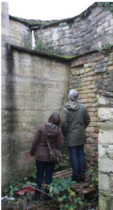
Historic England assess the Bastion interior.
