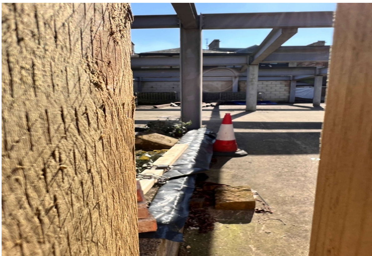
Site view inside hoarding from North Street
