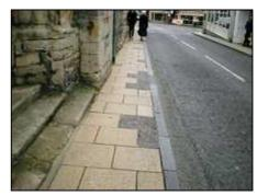
14. High Street St Martin's: junction with Kettering Road, north side; five or six kerbstones missing, tarmacked with two different types and some remains of pebbled concrete; no indication of kerb edge making it extremely unsightly and dangerous for pedestrians. It needs new kerbstones and to be re-covered with paving slabs to match those existing.
