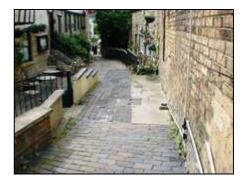
**5. All Saints Street**: cross-over access to the Brewery is in very poor condition, patched with concrete and other materials. This is a high profile site in the town centre and needs to be replaced with granite blocks to blend with the Brewery forecourt.
