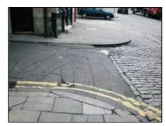
**7. Broad Street:** north side, adjoining Nos. 6-8; the pavement grouting is of very poor quality, plus pre-cast slabs used in places – it needs to be re-grouted and the concrete slabs replaced with proper paving slabs.
