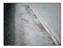
**2. King's Mill Lane:** tarmac at the junction spills over from St. Peter's Street – this should be replaced with matching granite blocks to blend in to the existing surface in King's Mill Lane. (Several of the blocks are covered with tarmac).
