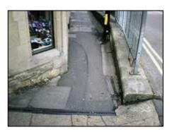
**4. Old Barn Passage**: there is a mix of materials used in this important historic footpath; the path has been patched up over the years using a variety of materials. This needs to be resurfaced with a consistent use of materials (e.g. granite blocks, paving slabs).
