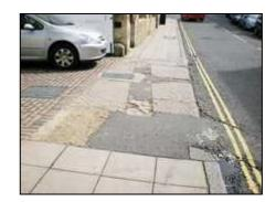
**6. Crown Street:** at junction with All Saints Place - access to pedestrian crossover is crudely executed with a tarmac ramp to the kerbstone. It should be re-laid to a higher standard and with a properly graded slope to street level.
