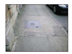
11. St Mary's Street: near to item10 above; the concrete surround to the fire hydrant needs to be replaced with paving slabs.
