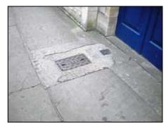
**12. St Mary's Street:** opposite St Mary's Church at the entrance to Stamford Walk; very poor quality repairs to the surface with a mix of materials, with four service covers in this small area. This should be replaced with granite blocks.
