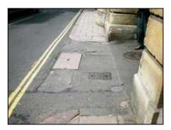
**13. St John's Street:** east side adjoining church wall; fourteen places where paving slabs have been replaced with tarmac, the paving slabs need reinstating.
