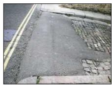
**3. Castle Street:** adjoining Paul Richman and near Bugle Lane; poor appearance in a sensitive area – the pavement is tarmac for c.6m and needs to replaced with slabs to blend in with the nearby slab surface.
