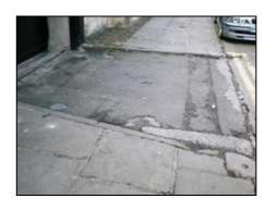
**9. High Street:** east end near Marks and Spencer; large area where the bricks have been replaced with concrete filler – the bricks need to be reinstated.
