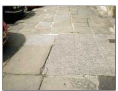
**8. Broad Street:** south side at No. 32 crossover access to private garage; poor quality patchwork of tarmac and concrete needs to be re-surfaced with a consistent use of material (e.g. granite blocks).
