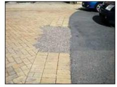
**10. St Mary's Street:** outside the Arts Centre; the surface needs to be replaced around the BT cover with paving slabs (as far as possible) consistent with the rest of the pavement.
