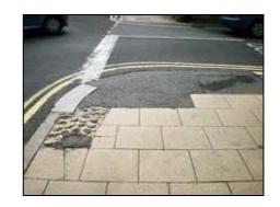
**15. High Street St Martin's:** south side; concrete and tarmac needs replacing with paving slabs as above.
