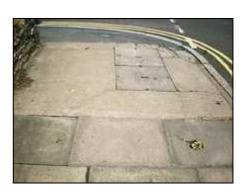
**16. High Street St Martin's:** junction with Barnack Road, south side; two or three kerbstones missing and missing paving slabs replaced by tarmac, paving slabs and kerbstones need re-instating.
